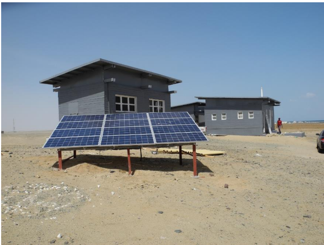
Figure 4: WCGA headquarters which were renovated during 2016-2017 (Photo R. Klaus).
